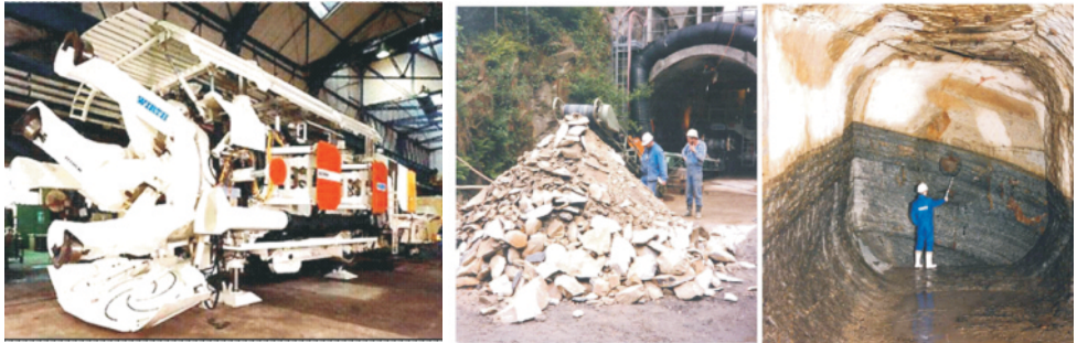
Fig. 6. view of the Wirth machine used undercutting method and the effects of its work
