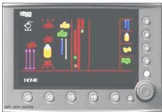
Fig 7. Bolting control panel
